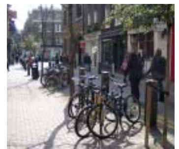
Stands placed at 45° to provide a clear path for pedestrians
