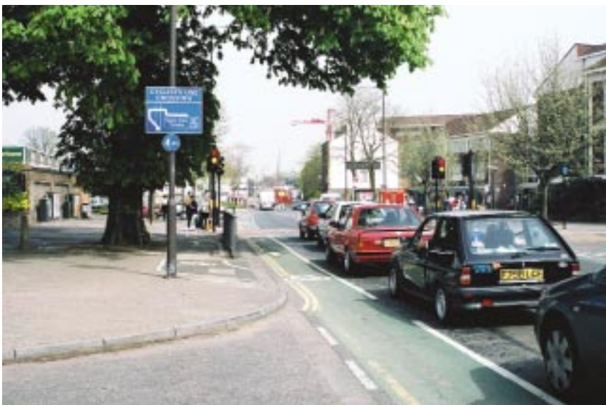
Exit ramp enables cyclists to use crossing to turn right across a busy road into Syon Park
