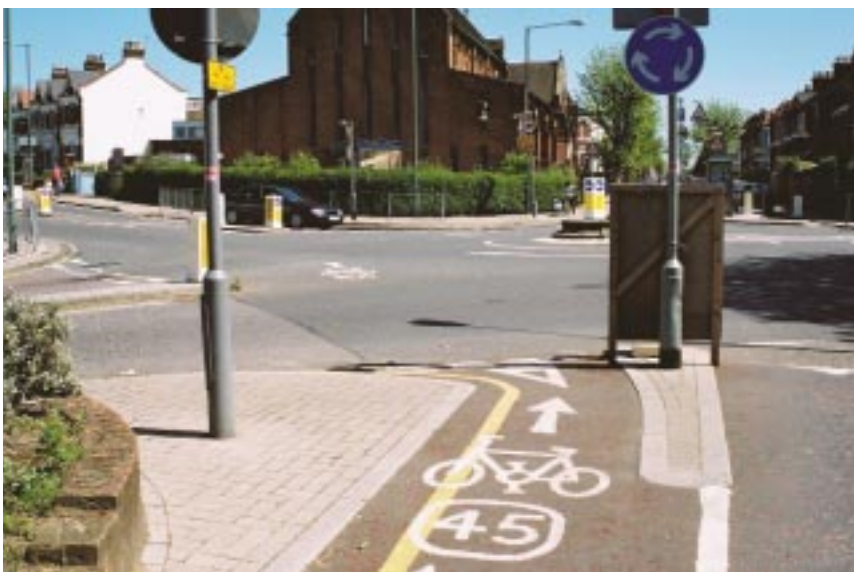
This contraflow cycle lane entry to a small roundabout works well
