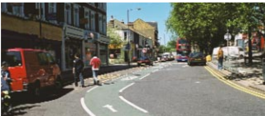
Take cycle lane outside bus stop cage and adjacent car parking where this can safely be achieved
