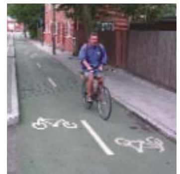
Use of broken white centreline and cycle symbols shows that facility is 2-way
