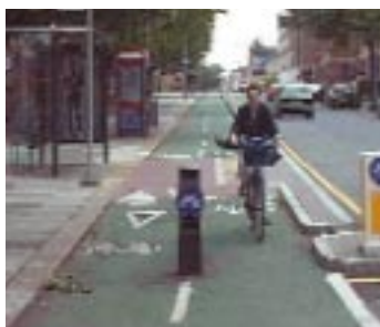
A table helps to slow cyclists at point of conflict with pedestrians
