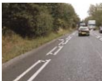
Hatched marking outside cycle lane
