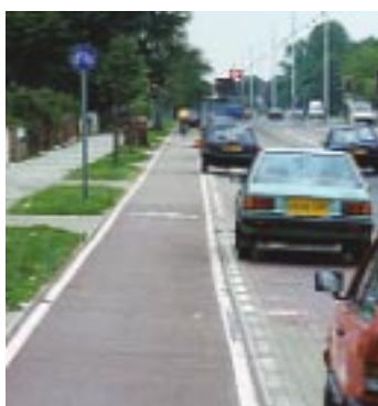
Lanes inside car parking offer cyclists good protection from fast traffic
