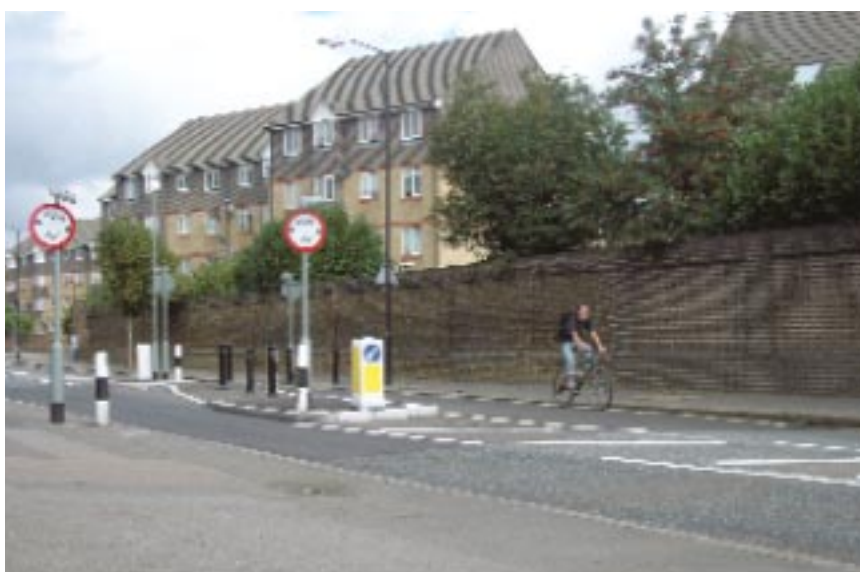
Horizontal traffic calming measures are usually more effective and comfortable for cyclists than humps
