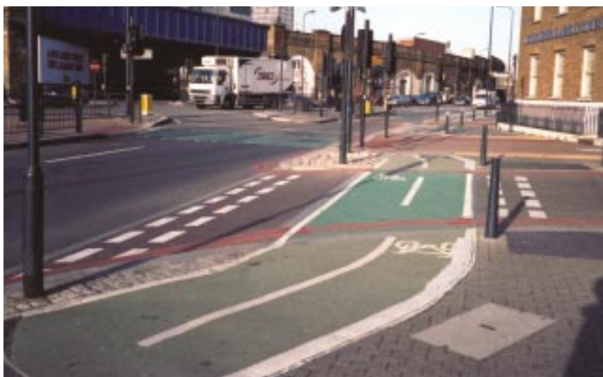
A well designed entry treatment will enable cyclists to maintain priority over side roads
